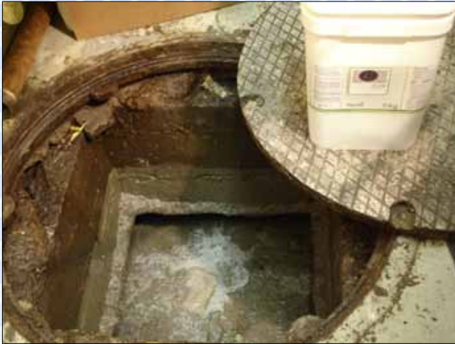
Initial stage of BCP10 application in wastewater system access.
